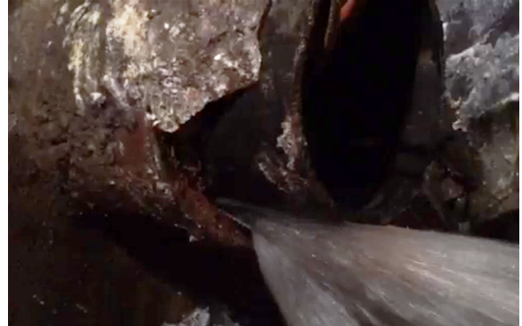
This still image from an on-site video shows the severity of the leaks.
